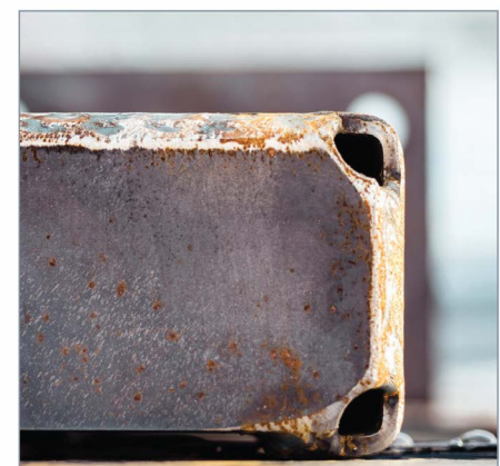
END PLATE VENTING. This is how a hollow section end plate should be cropped at all corners prior to attaching to prevent zinc and air traps.
